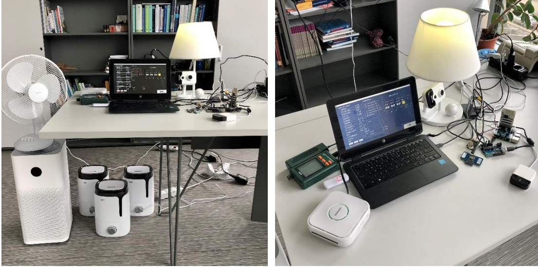
Fig. 5. The installed equipment of the REACT system
